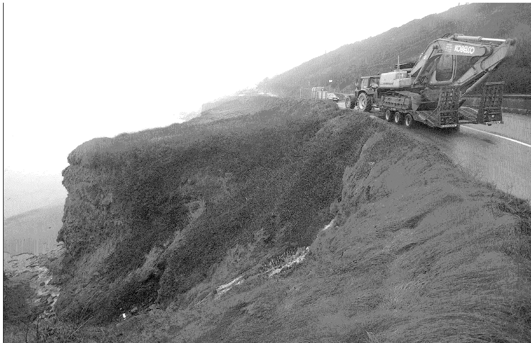
The road along Inch strand on the Castlemaine-Annascaul road in Co Kerry, which is under threat from coastal erosion. Photograph: Don MacMonagle
