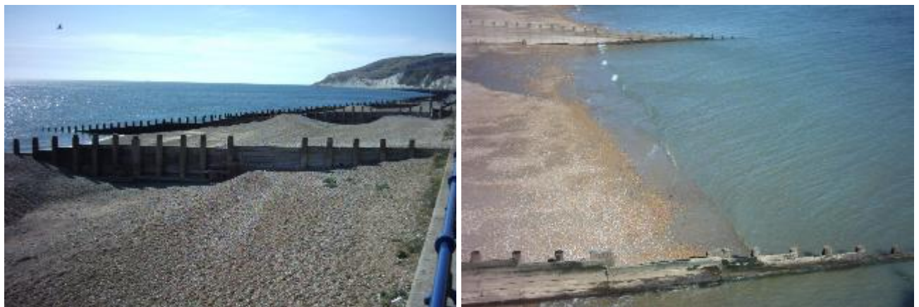
Figure 32 Timber groynes at gravel beach of Eastbourne, East Sussex, UK
