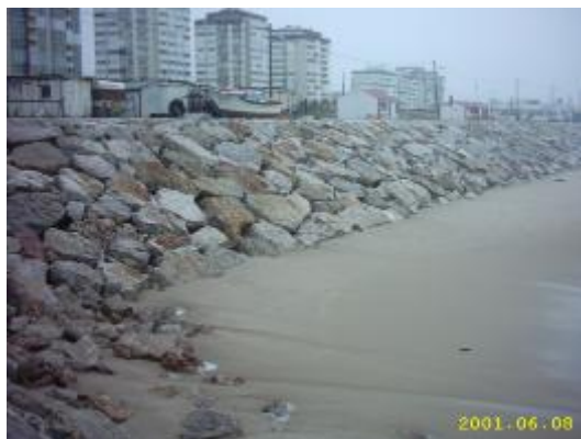
Figure 26 Coastal revetments and groynes at Caparica, South of Lisbon, Portugal
